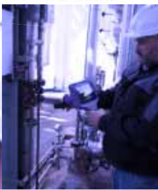
STEAM TRAP INSPECTION
